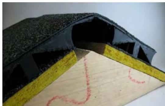
Figure 3. The end of this ridge vent is open to wildlife entry. Photo by Stephen M. Vantassel.
