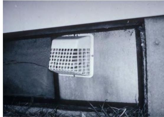
Figure 12. Plastic vent cover suitable for bathroom exhaust vents.
