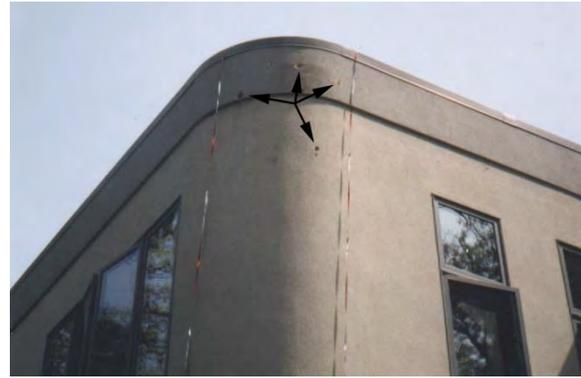
Figure 6. Arrows point to downy woodpecker holes in the synthetic stucco. The vertical lines are Mylar® tape installed when the damage began. Photo by Stephen M. Vantassel.
