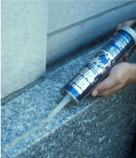
Figure 19. A polybutene-based product being applied to a ledge to repel birds. Photo courtesy of UNL.
