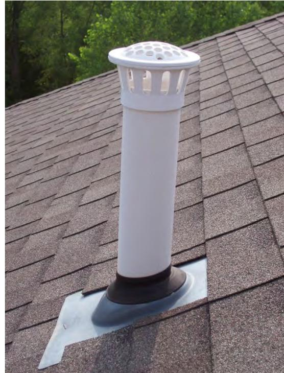
Figure 13. Sewer vent pipe cover.
