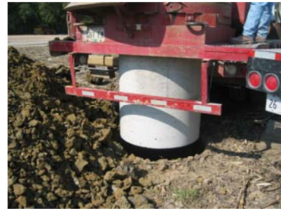
setting casing into hole
