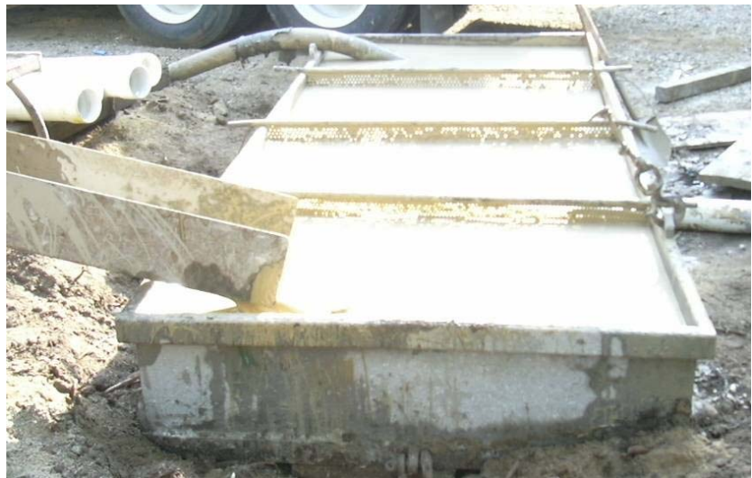
A typical above ground mud pit:
