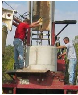
setting casing through the ring gear
